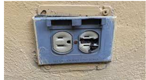
Damaged Outlet
