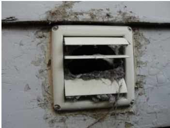
Broken/Clogged Vent
